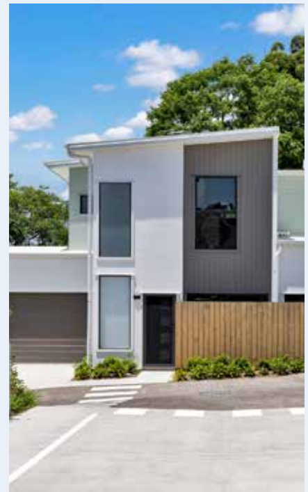
Front façade of townhouse located in Bellfield Terraces, Aspley, QLD
