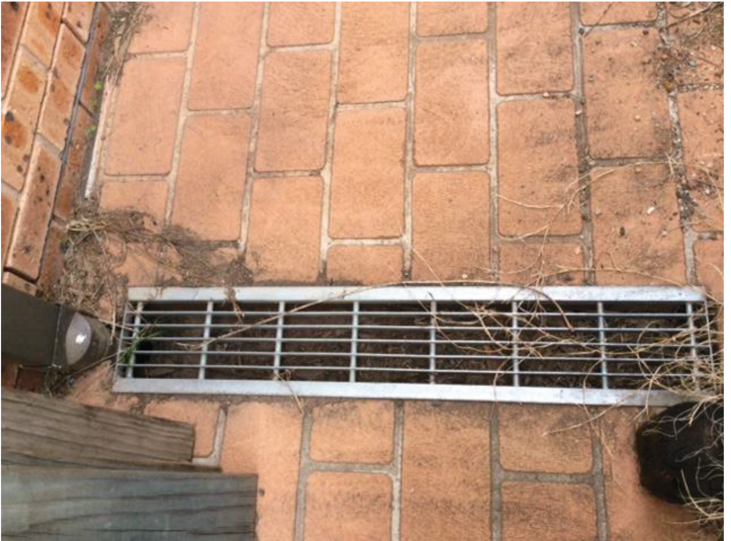
Channel strip drain across path between laundry and rear of house
