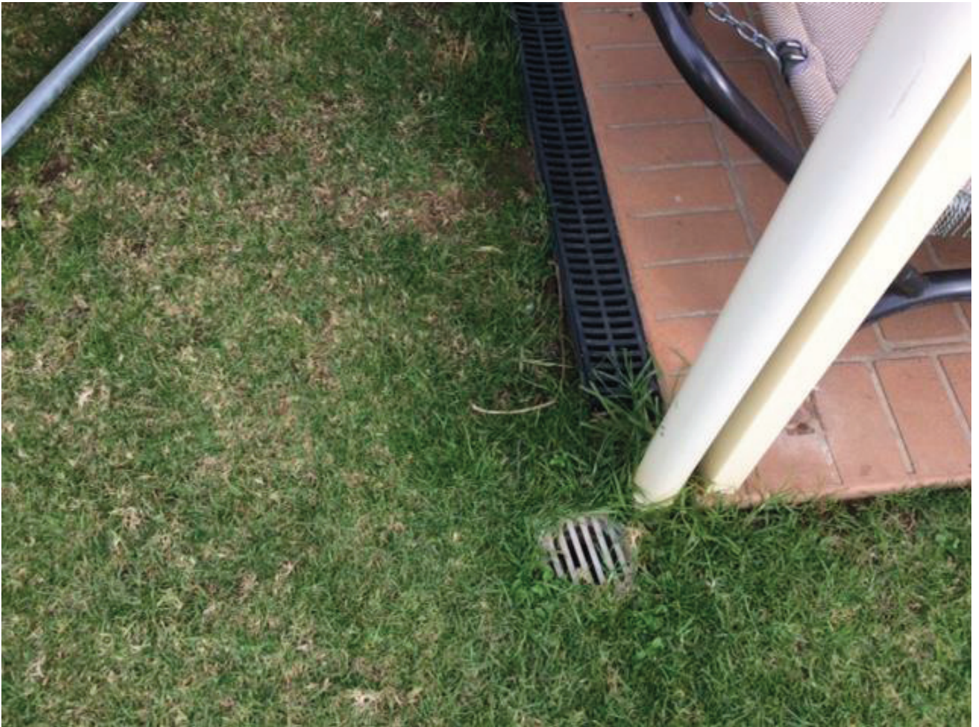
Surface drain and the new channel strip drain installed alongside pergola.
