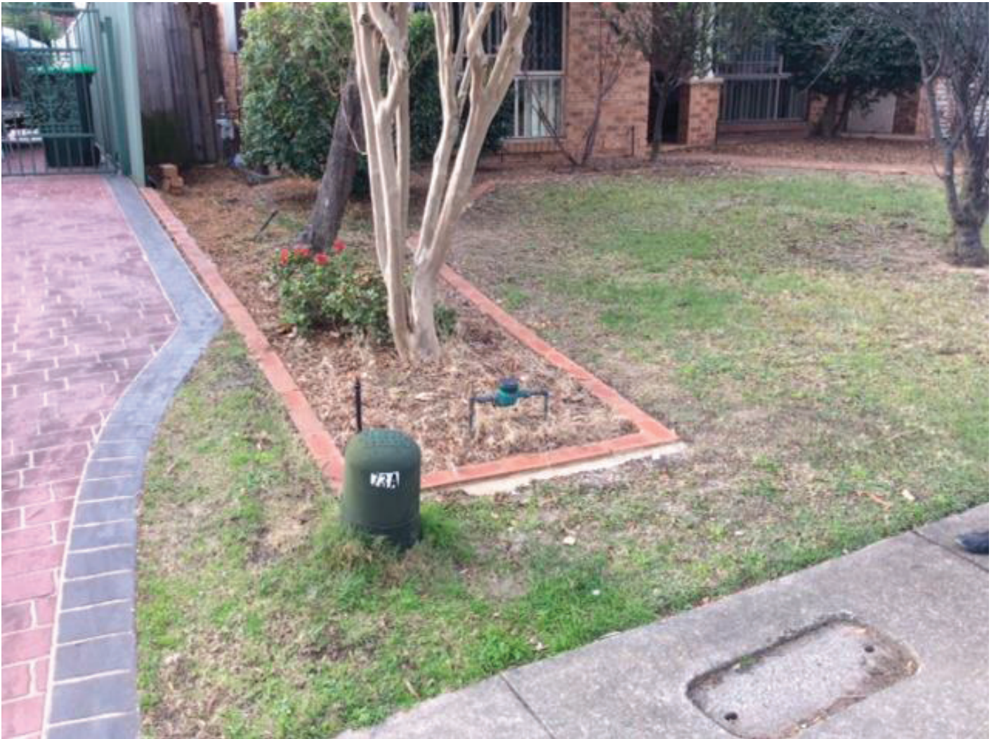
Services corridor contains, gas, water, phone and power. Stormwater exits at street kerb beyond Telstra pit.
