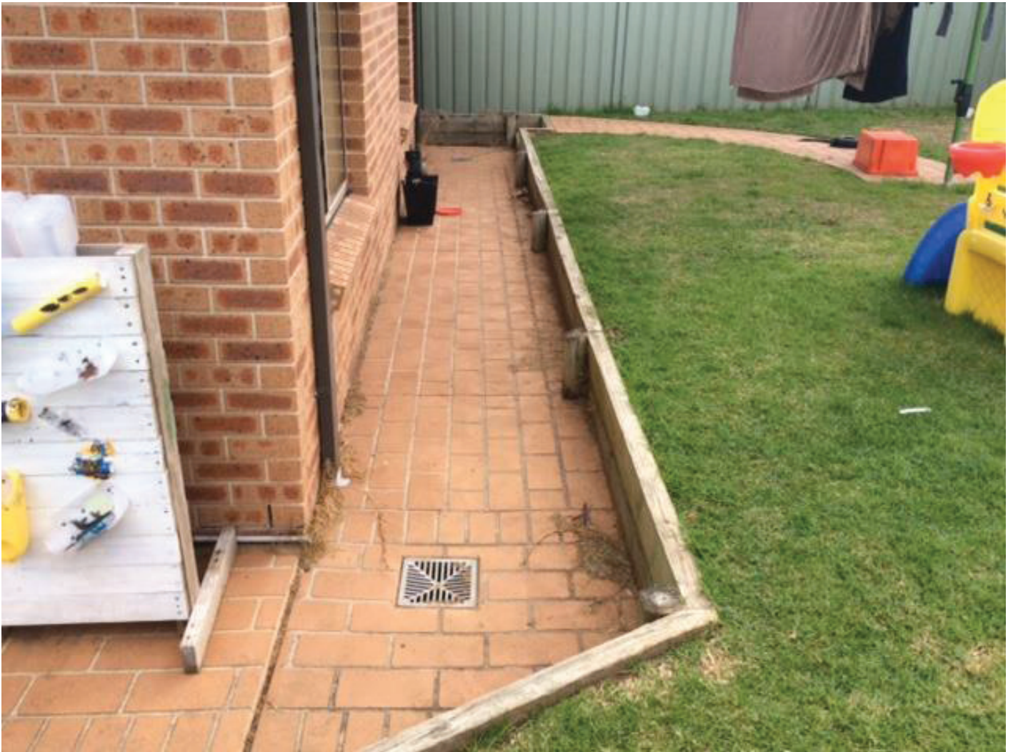
Two 200x200mm stormwater pits located in path at rear of the house below the retaining wall
