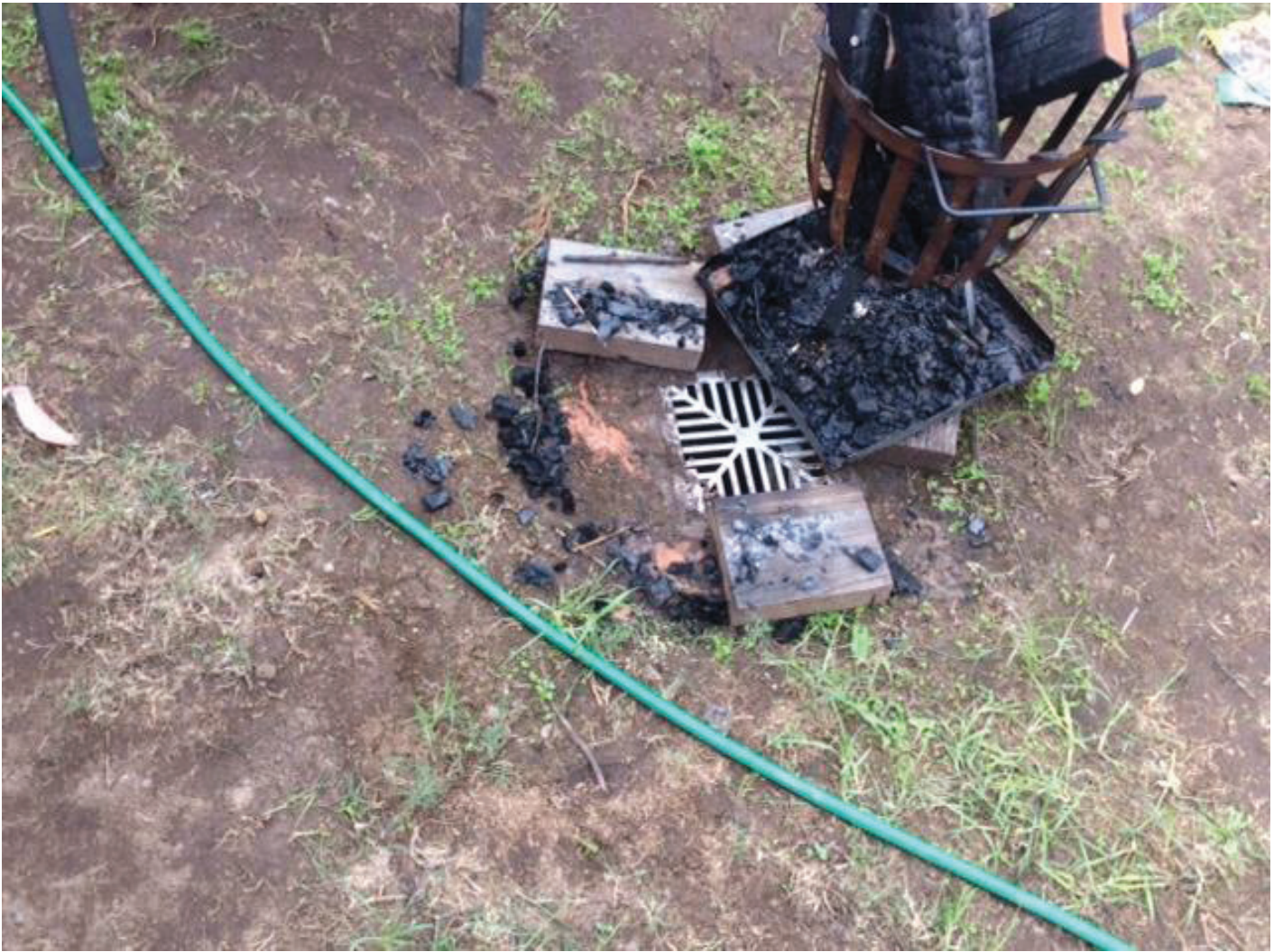
Additional stormwater pit in rear yard between pergola and right side fence
