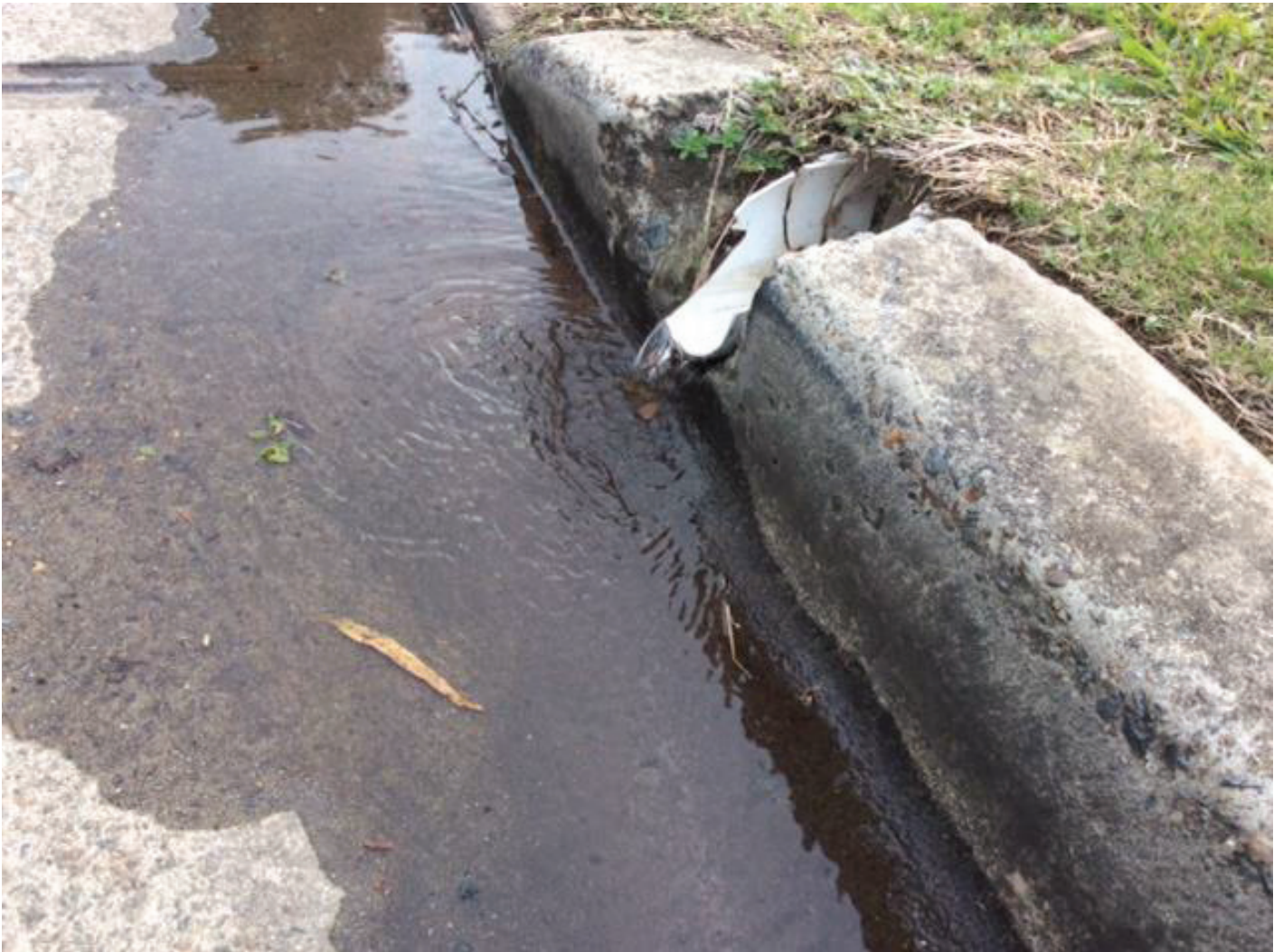
Good water flow at street kerb and equals the hose putting water into the system
