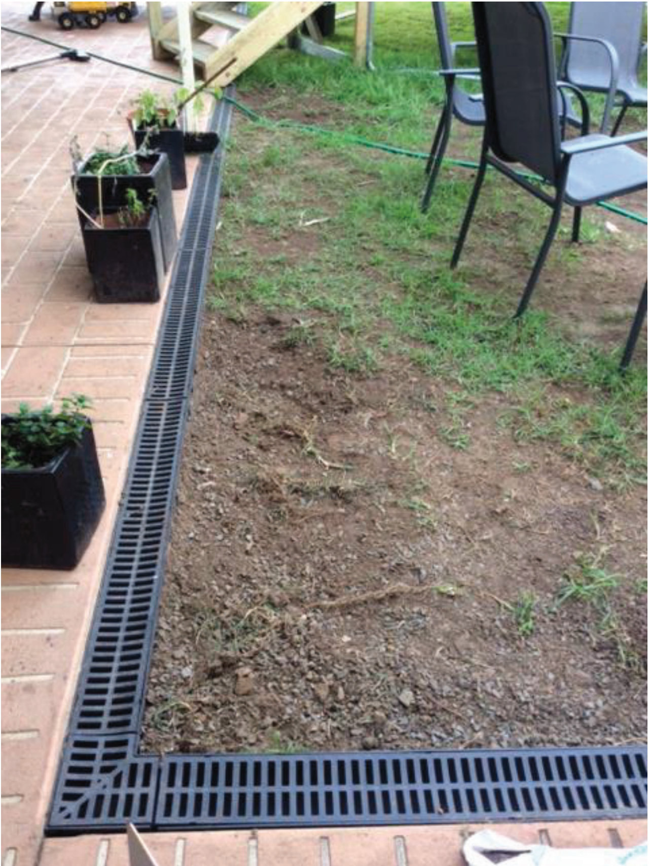
New channel strip drain installed across rear of garage and runs alongside pergola – looking alongside pergola. Note damage by tenants dog
