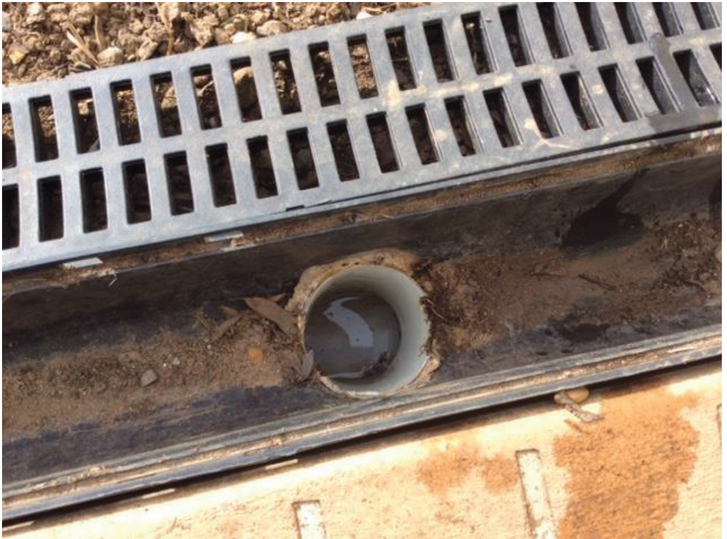
The channel strip drain installed at the rear of the garage.
