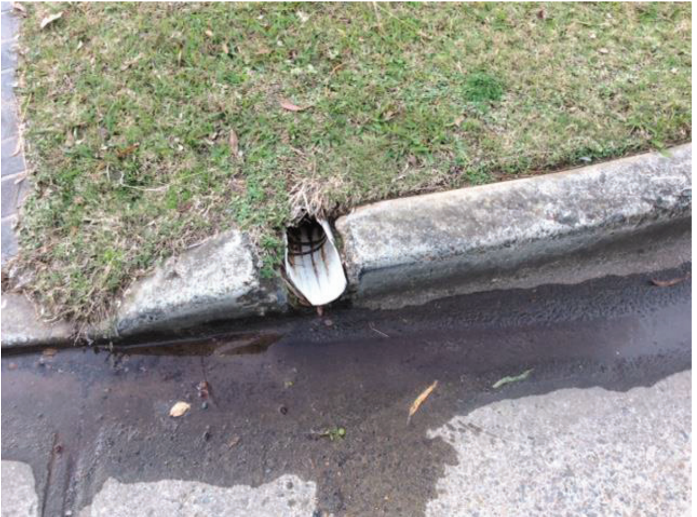
Water exits the street kerb after 14 minutes of filling the stormwater system.
