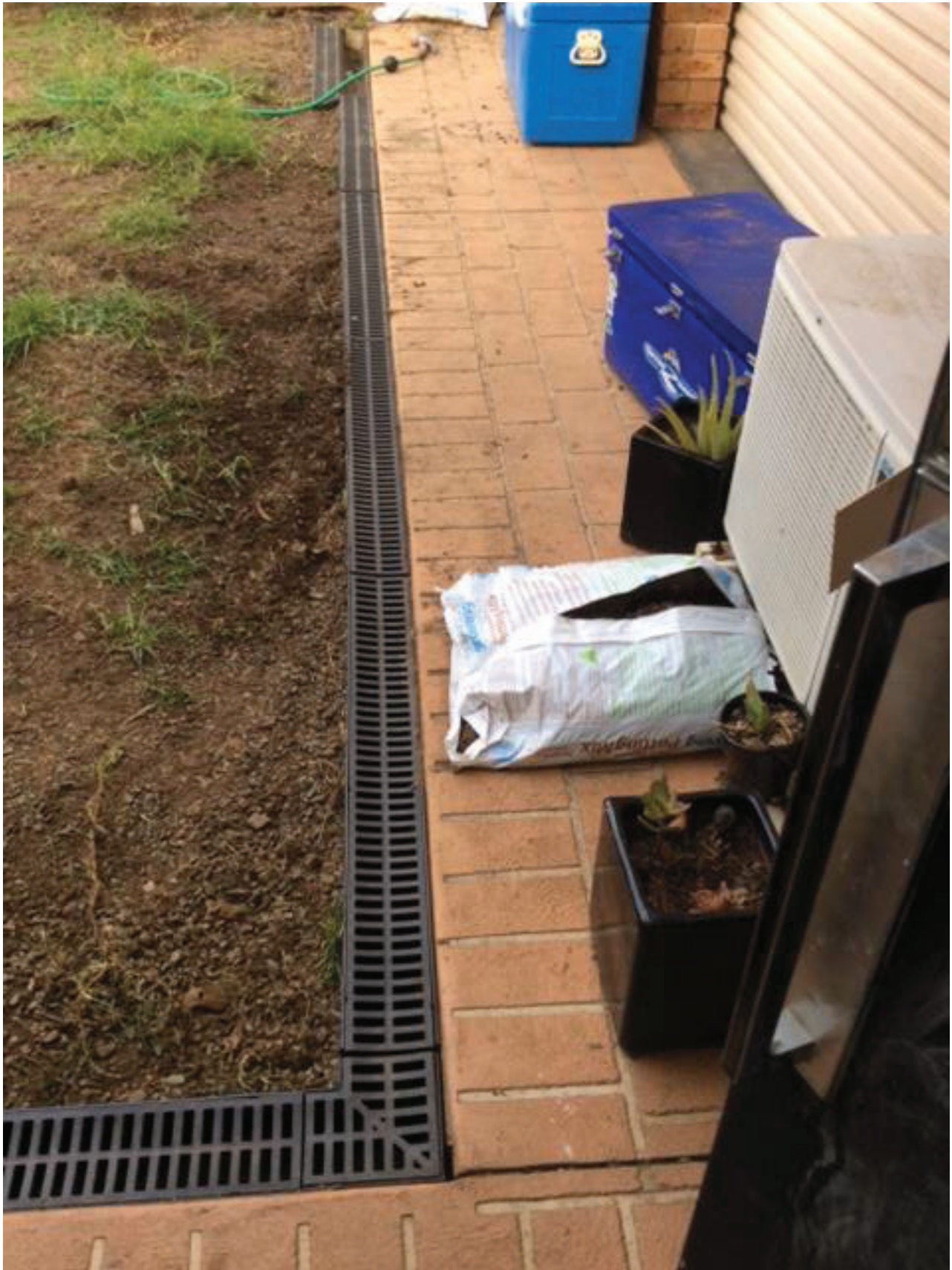
New channel strip drain installed across rear of garage and runs alongside pergola – looking across rear of garage. Note damage by tenants dog
