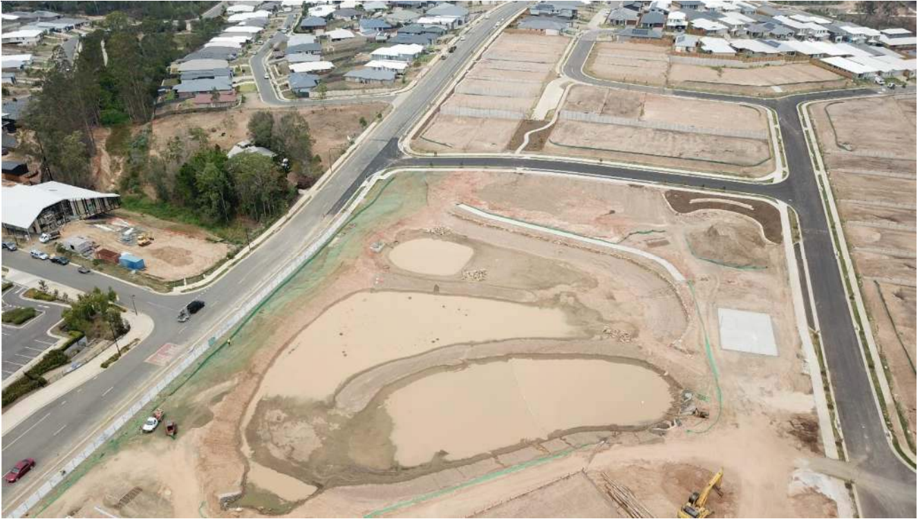
Photo 1: Aerial view of Stage 2 Wetland Construction– December 2019
