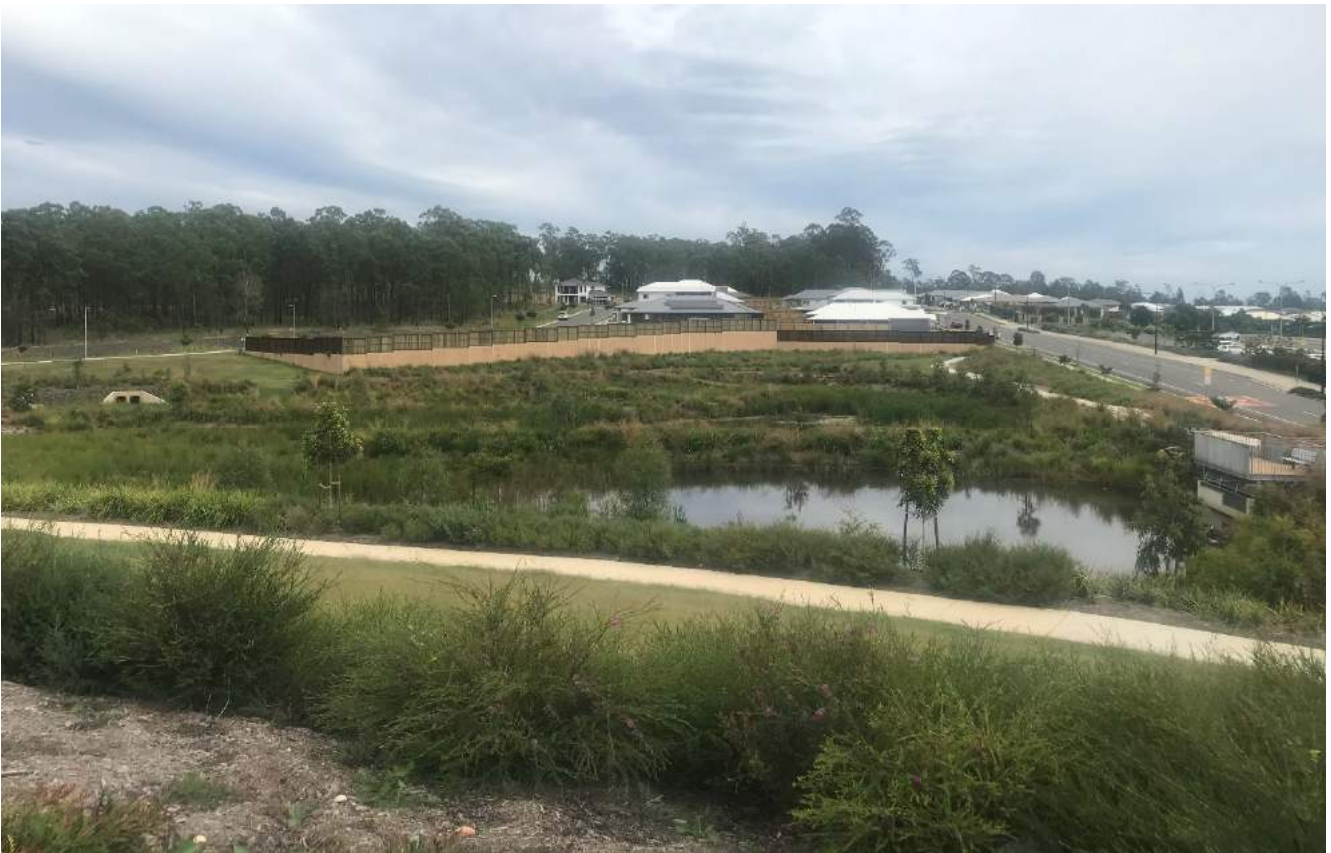
Photo 2: Stage 2 Wetland Construction – April 2021
